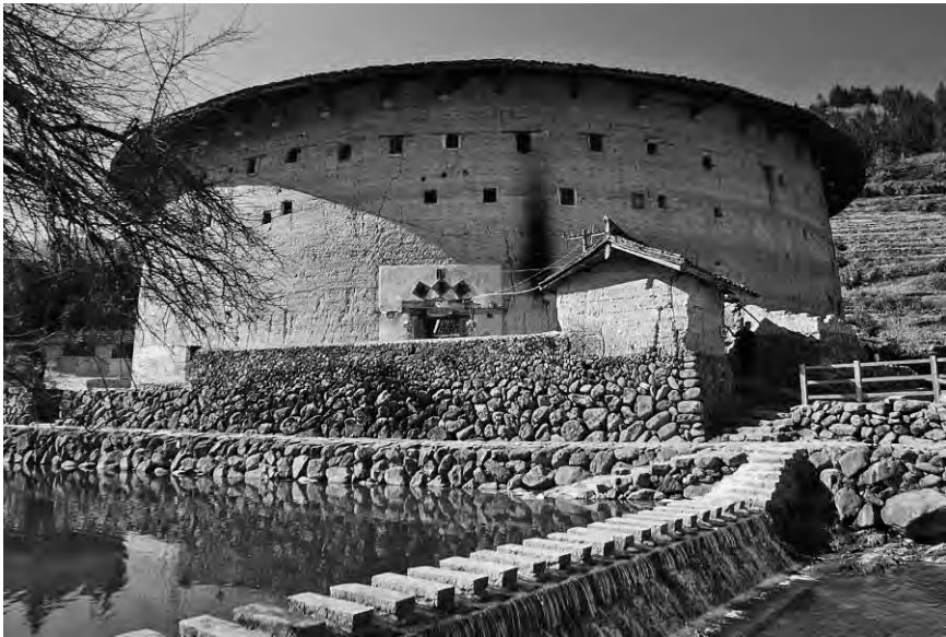
1.1 Yuchang Lou in Fujian, China: a wood–clay composite building that is over 600 years old.
