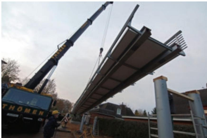
Figure 10: The Holländer Bridge in Germany uses Fiberline pultruded decks in conjunction with steel beams.
