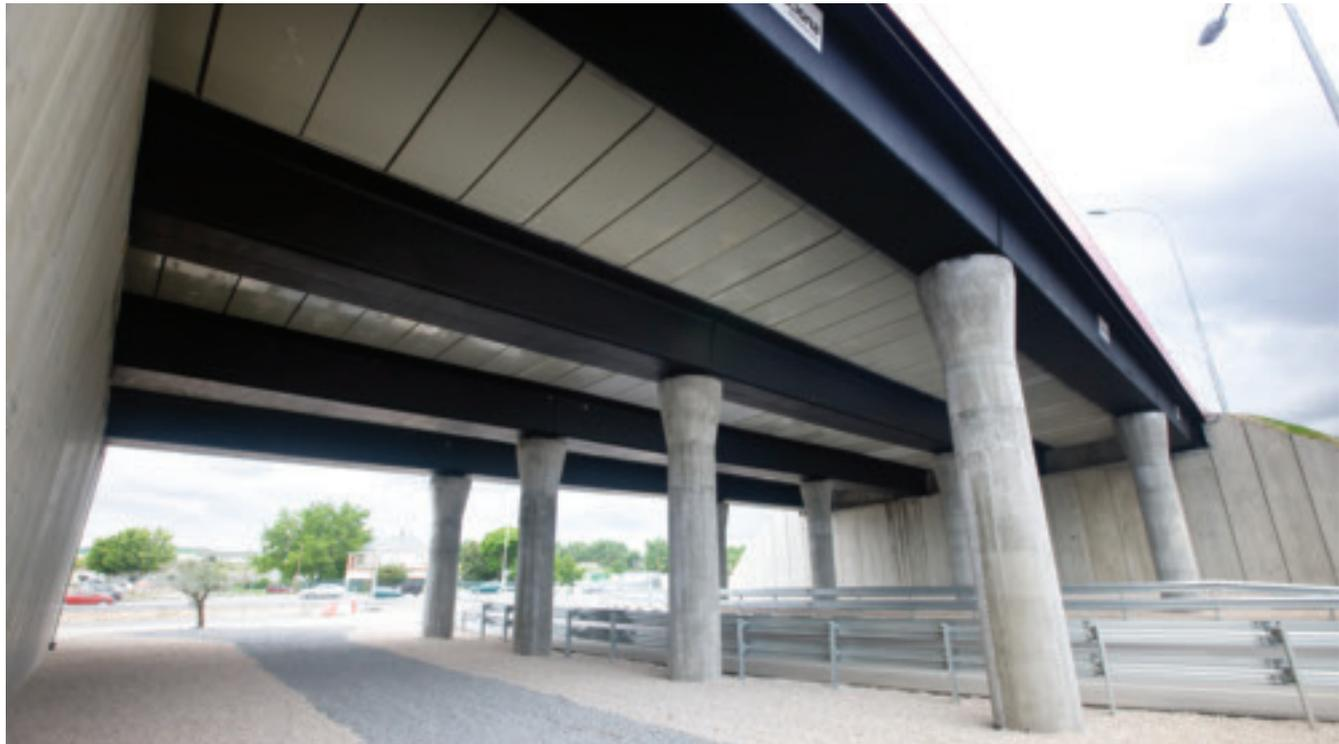
Figure 8: Road bridge in Spain produced by Acciona Infraestructuras, consisting of moulded FRP primary beams and concrete decks.
