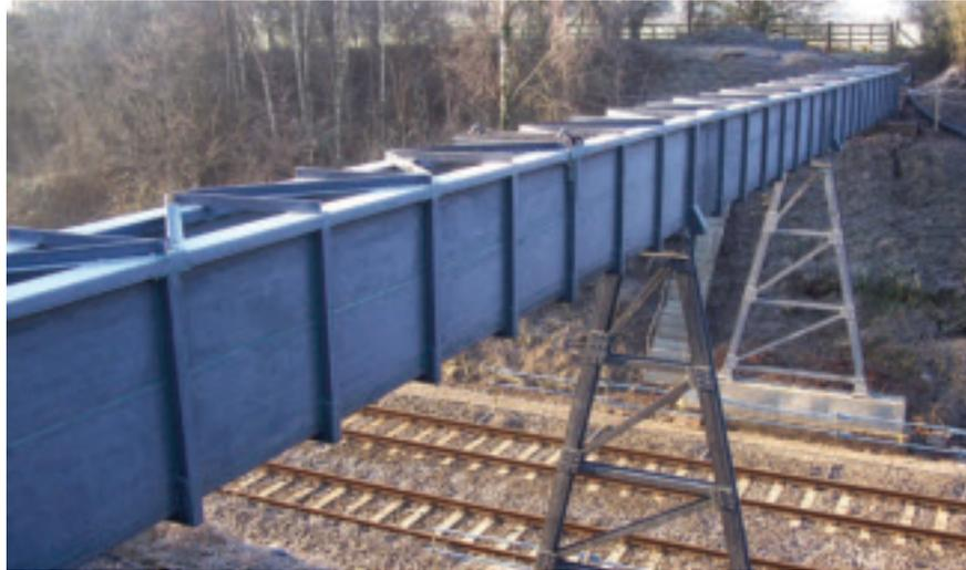
Figure 9: Launder Aqueduct fabricated from pultruded panels.
