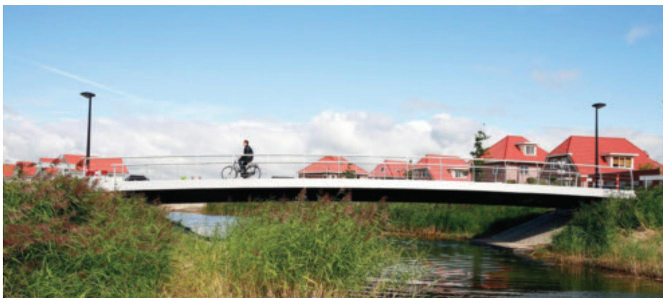
Figure 7: Carbon FRP bridge produced by Fibercore, spanning 24.5 m.
