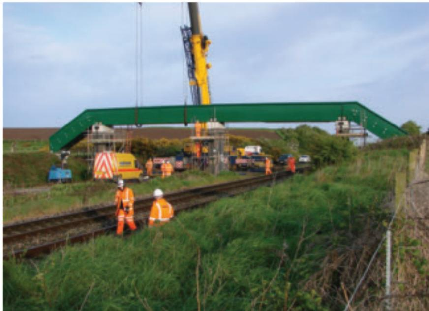
Figure 2: Bradkirk FRP footbridge. (Picture courtesy of Birse Rail.)
