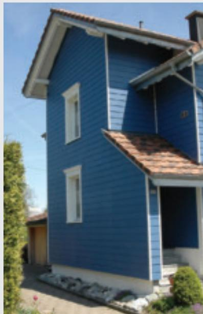
**This house was built using Tech-Wood's WPC siding, developed in cooperation with extruder manufacturer Cincinnati Extrusion.**
