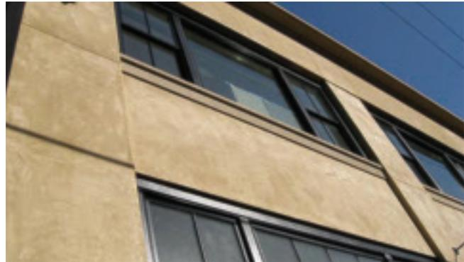
*Simulated stone exterior trim features a polymer concrete face coat backed with FRP sheets on this Kreysler project.*
