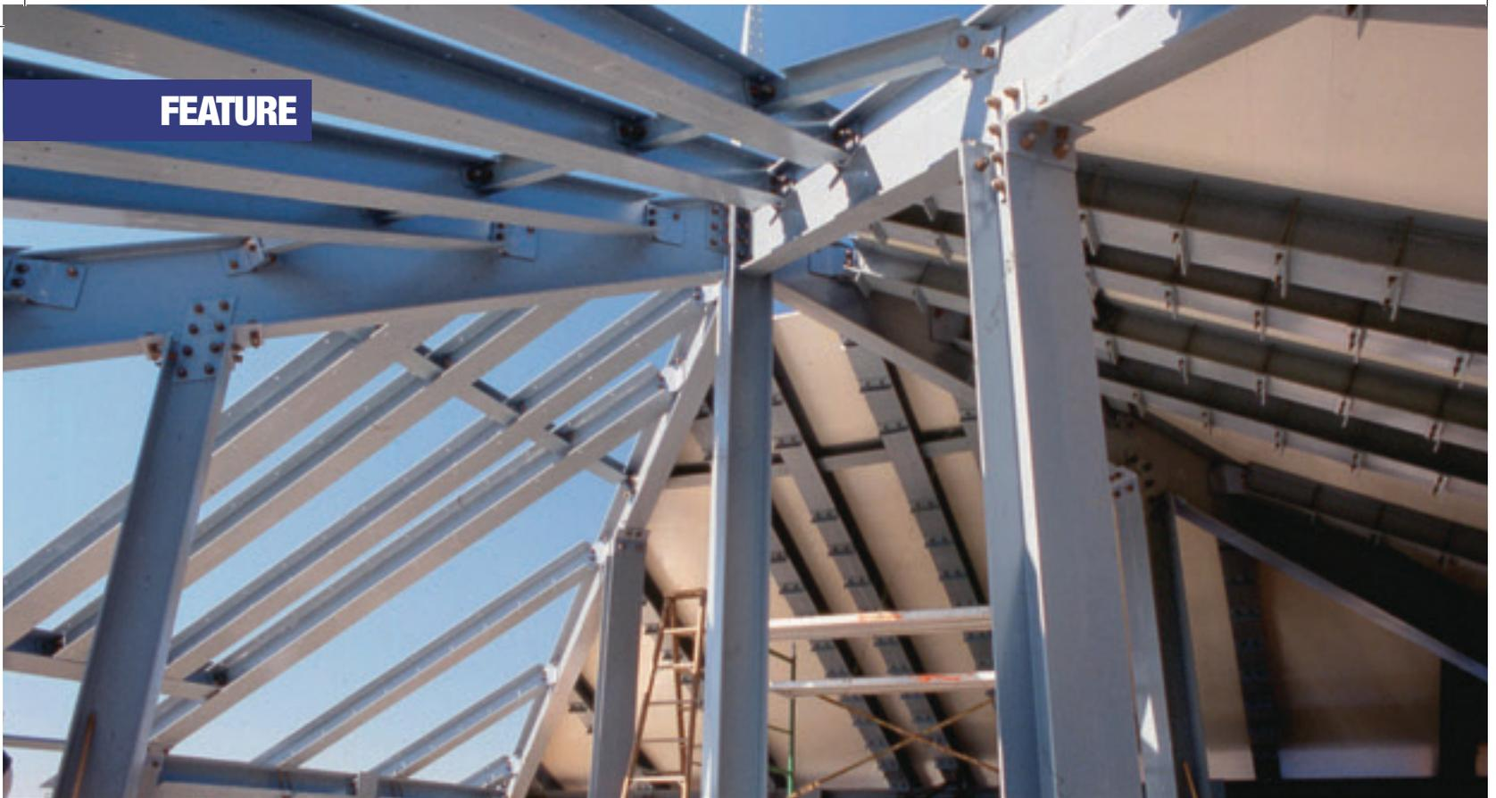
*Strongwell's Extren® structural beams were selected for this technology building because the FRP material does not block radio frequency waves.*
