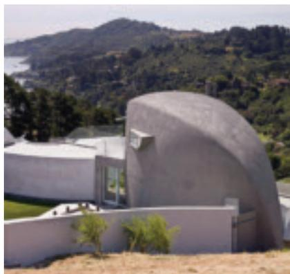
**Kreysler's award-winning California Bay House is a monocoque structure consisting of nine custom-moulded, fire-retardant FRP sandwich panels.**
